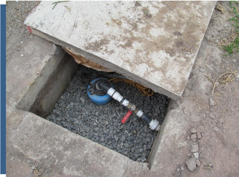
Pictured: the finished top of the borehole
