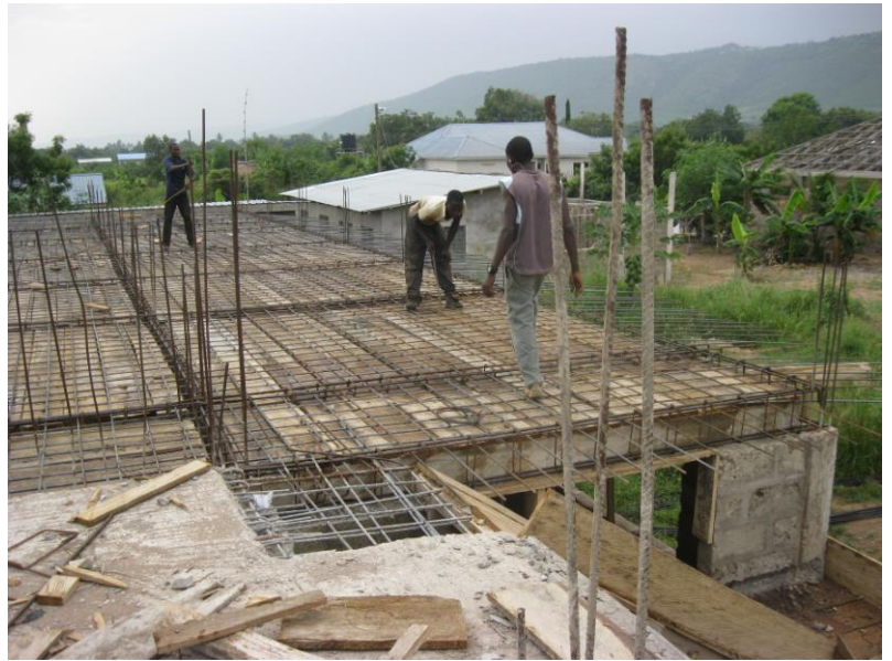
casting the roof in early January 2013
