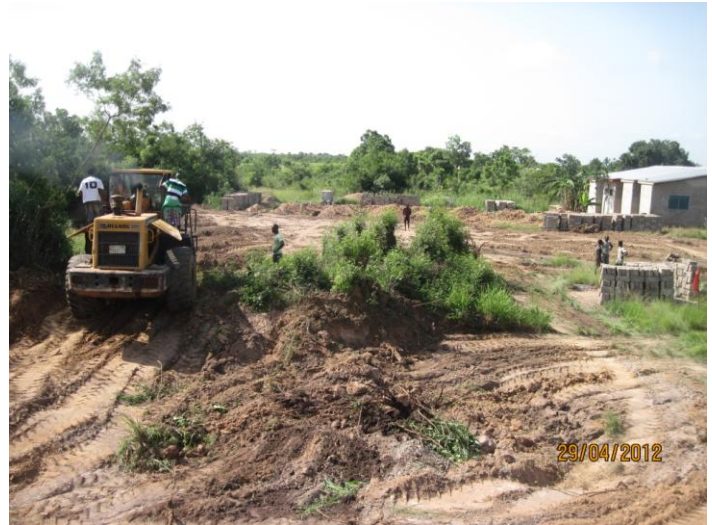
A bulldozer levels the plot recently attained by MOP
