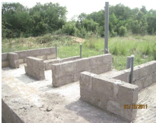
the future boys' bathroom with 2 showers (left) and 2 toilets (right)
