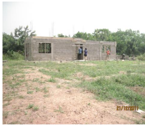
the front room at Ayikuma completed up to ceiling level.
