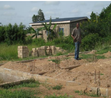
Eric Kwame Agoe stands on the finished foundation inspecting the filling.
