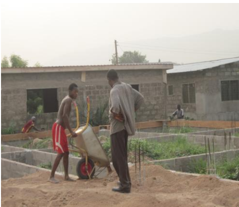
Spring 2011 community members & volunteers worked together filling the building foundation.
