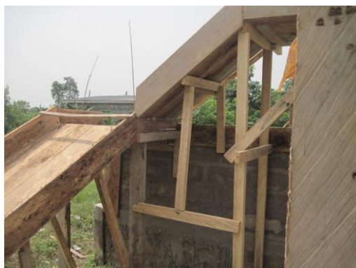
Staircase leading to second story
